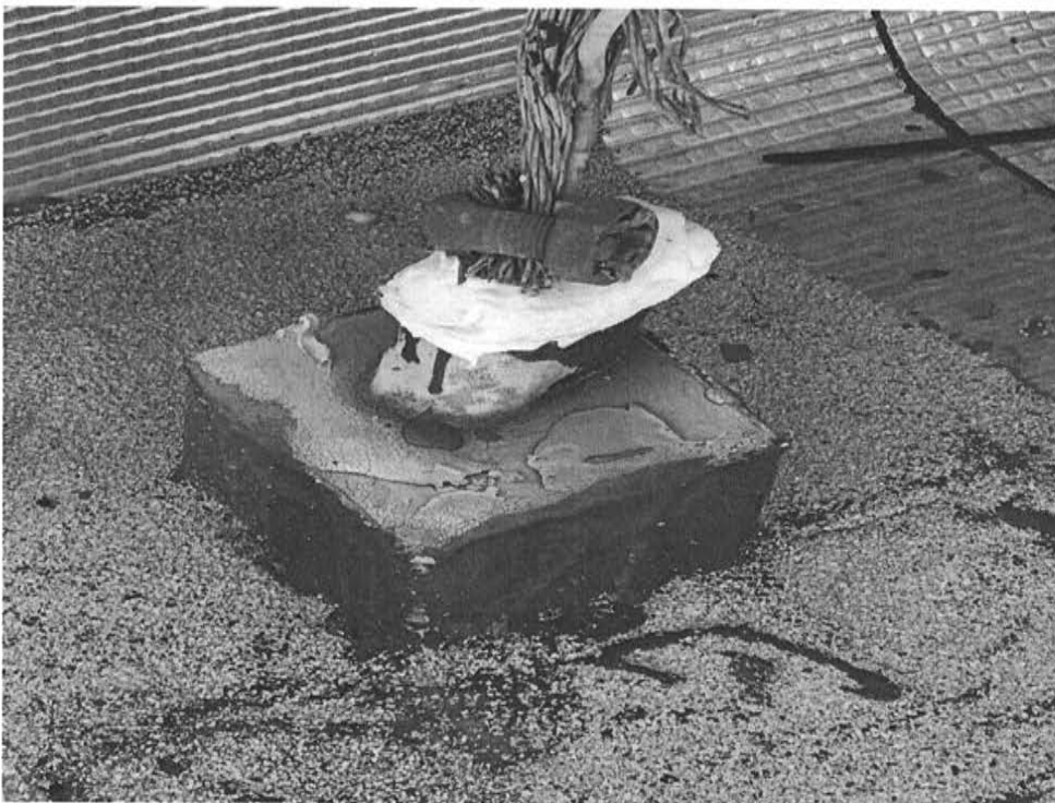
Photograph No.2- Close up of ultraviolet damaged pan filler.
